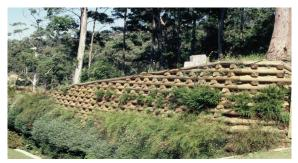
The Log Crib has been designed to provide an attractive, easy to build structural retaining wall system where ground conditions are unsuitable for deep post embedment and where top soil conditions are suitable for the crib type of structure.
