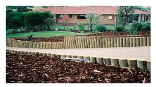
• This type of wall is a variation of the Closed Face Cantilever Wall and the construction methods are basically the same except that a continuous trench is dug rather than individual post holes. Any naturally occurring taper can be compensated for by alternating thick and thin ends. To provide stability and hold alignment of posts in high walls during setting, use wire and staples along the top of the posts. This can be removed on completion of the job.
